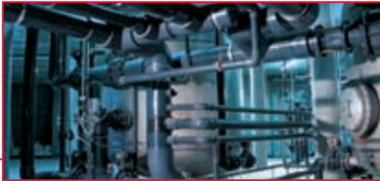
Water Purification Plant | Italy
